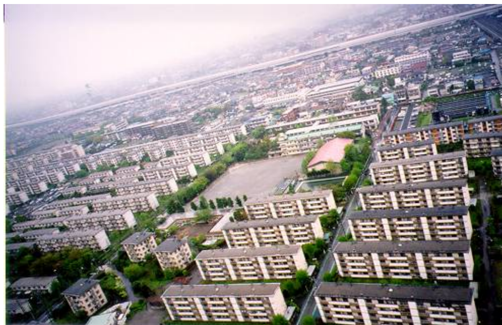
Soka Matsubara Danchi (housing complex)
