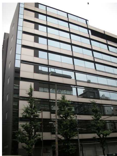
Photo 1: Exterior view of the new office
