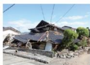
Photo 9-1 Collapse of wooden houses.
